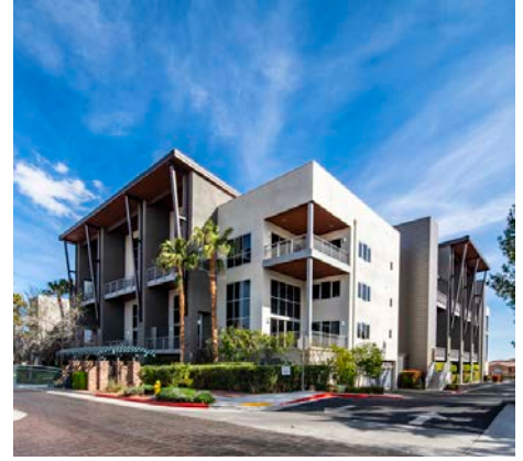
C2 Lofts and Parking Garage Las Vegas, Nevada 4-story, 2 Bldgs, 100 Units | New Construction Client: Christopher Homes *Experience of Adriana Gonorazky
