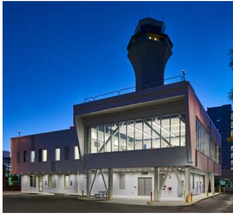
FAA Portland PDX Administration Building Portland, Oregon 10,000sf, 2-story | New Construction [Design-Build] Client: Wu Construction/Perez Architects
