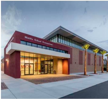
Las Vegas Day School Gymnasium Las Vegas, NV 16,000sf | New Construction Architect: Simpson Coulter Studio
