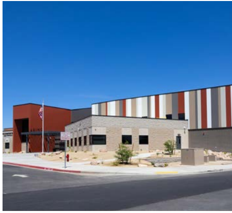
Clark County School District Laura Dearing Elementary School Las Vegas, Nevada 70,211sf, 2-story | New Construction Architect: KGA/PUNCH
