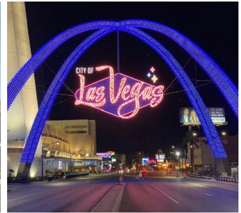
Las Vegas Arch Gateway Sign Las Vegas, Nevada Two, 80-foot arches supporting a 27' x 40' LED city logo, 30 feet above pavement Client: Yescos
